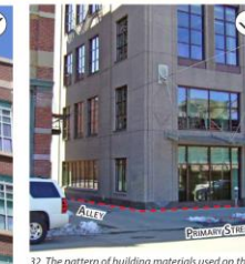
32. The pattern of building materials used on the Lower Story Facade shall continue around an alley corner onto approximately 25 feet of the lower stories of the Alley-facing Facade.
